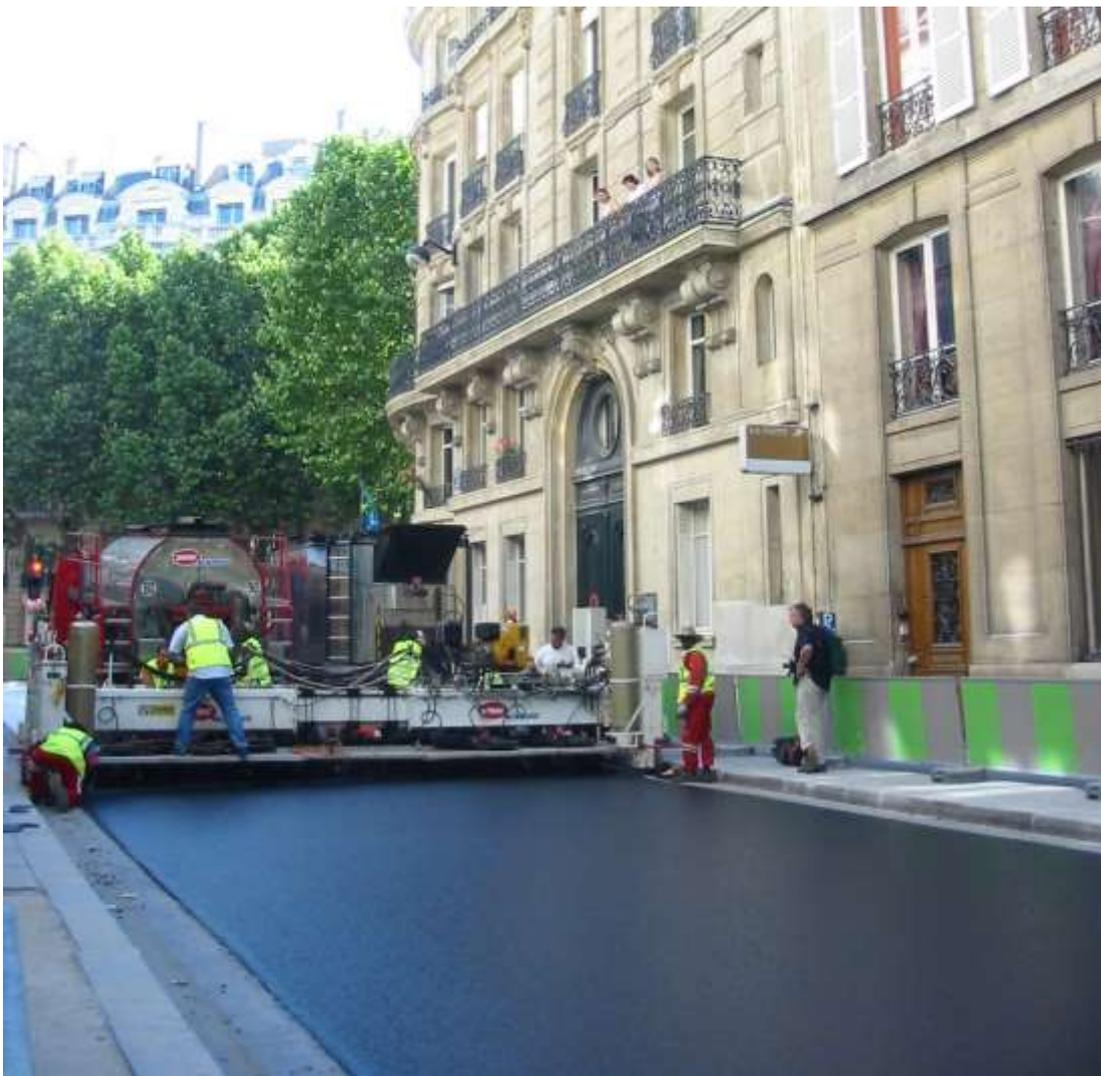
*Figure 8: Machine laid mastic asphalt pavement.*
