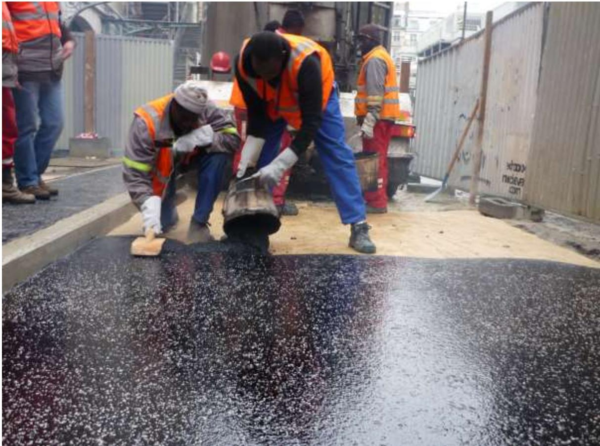
*Figure 7: Hand laid mastic asphalt screed.*
